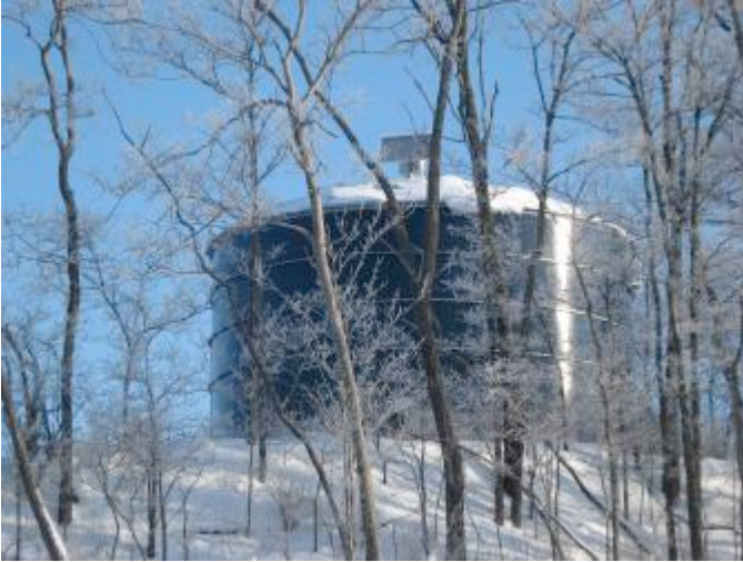
Figure 3. Bolted-steel reservoir with solar panels mounted on the roof to power a SolarBee mixer
