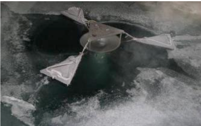
Figure 4. Holes can be broken through ice up to about 6 in. thick to install a SolarBee mixer.
