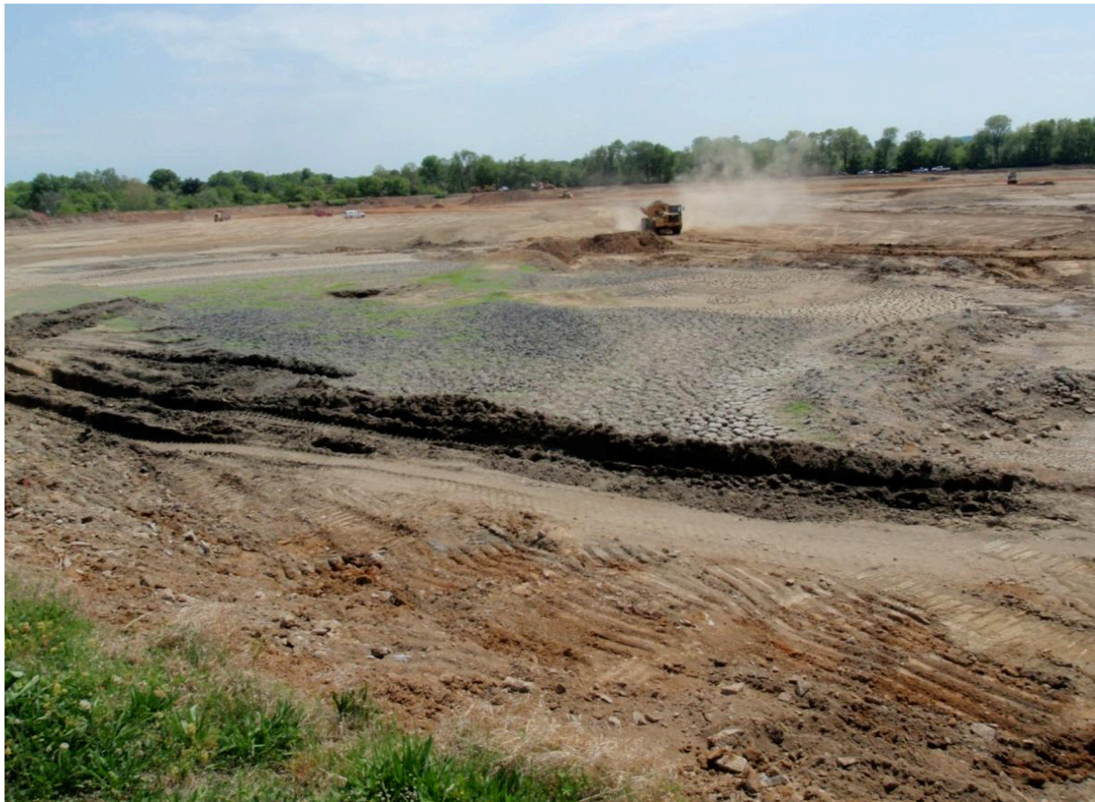
Figure 3: Disposal of filter backwash solids
