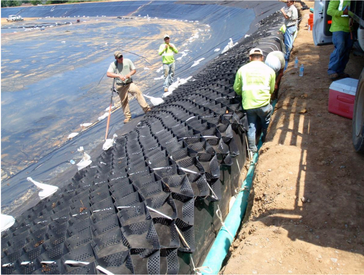
Figure 5: Installation of geoweb along the side slopes
