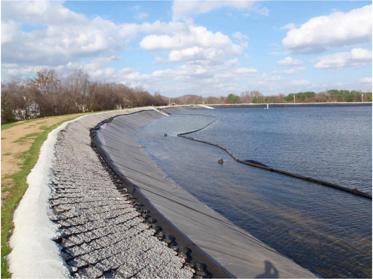
Figure 6: Completed reservoir rehabilitation shown now full of water
