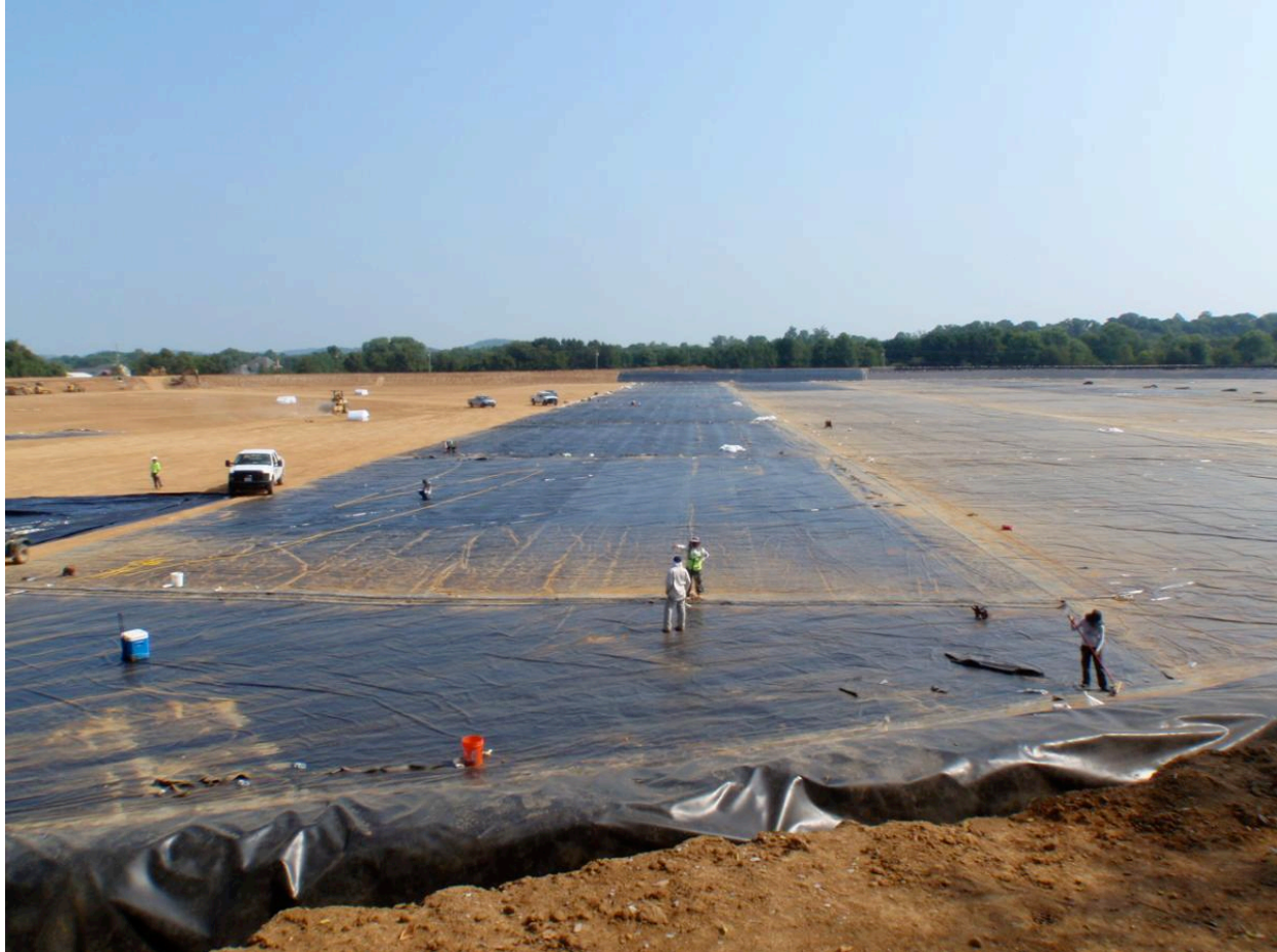
Figure 4: Geomembrane liner installation
