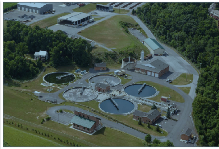
Figure 1. Aerial of Hampden Township's Roth Lane WWTP in Mechanicsburg, PA
