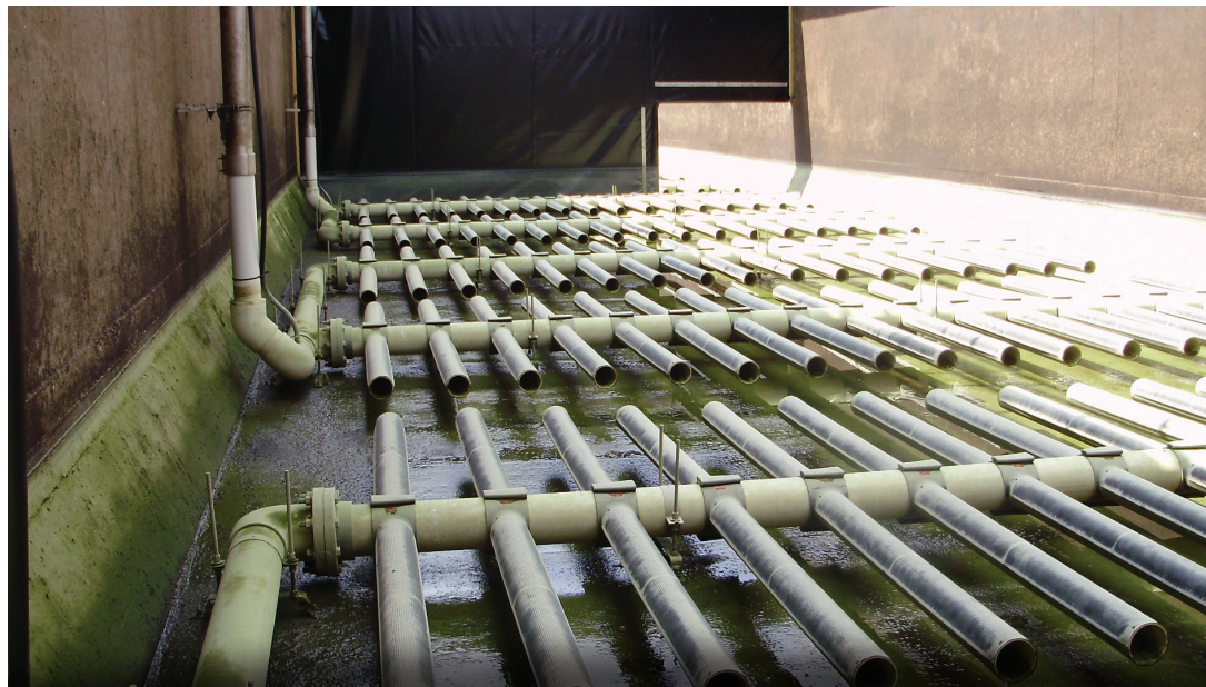
Installation of Mini-Panel Diffuser System
