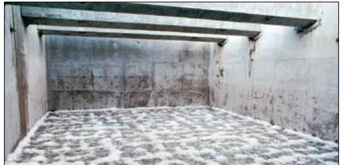
Better air scour action – and better media cleaning – is the result of closely spaced, non-clogging orifices and uniform distribution of air throughout the length of the underdrain lateral.
