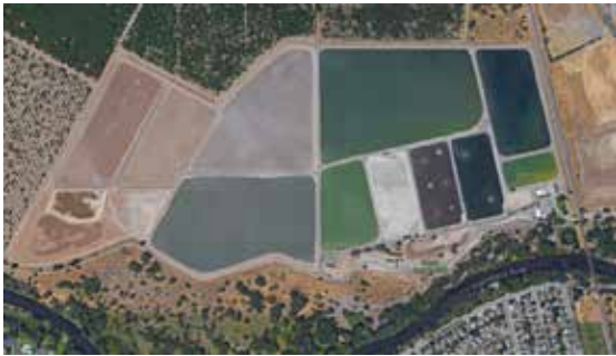
Figure 1: Wastewater Treatment Plan Aerial View
