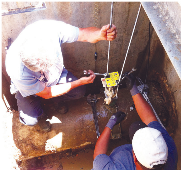
Figure 2: Installing insertion style mag meters such as the McCrometer FPI meter instead of Venturi and other full bore meters eliminates the need for line shutdowns, heavy equipment and extra labor costs.
