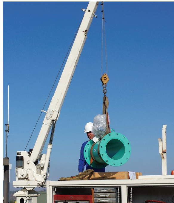
Figure 1: Installing a full-bore electromagnetic meter
