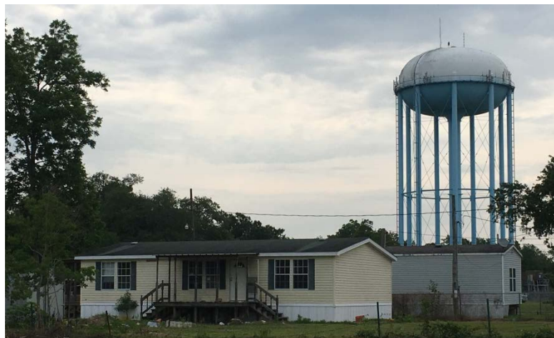
Figure 2: Water Storage Tank, New Orleans LA USA (PICK 1 OF 2)
