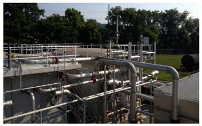
Figure 5: Membrane tanks of the AnMBR system at the confectionery manufacturing plant
