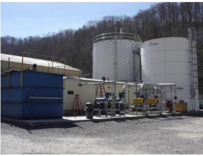
Figure 10: AnMBR + MBR wastewater treatment system at Kellogg Company Pikeville Plant
