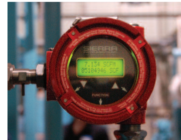
Sierra Steel-Mass™ 640S on a digester tank
