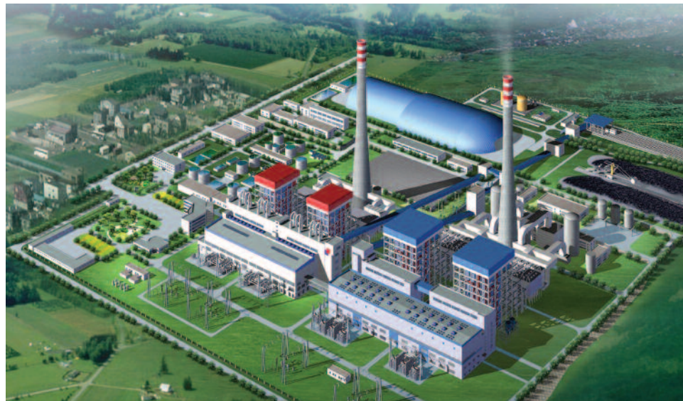
Yiyang coal-fired power plant in Yiyang, China
