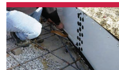
» Embedded Starter Used for larger municipal and industrial applications and higher seismic applications
