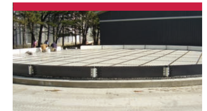
» Coated Steel Floors Glass-fused-to-steel and epoxy coated panels are bolted and sealed to cover floor surface
