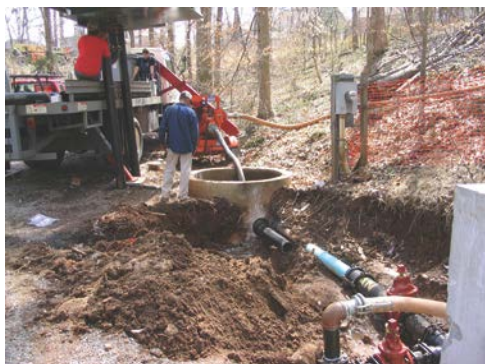
Figure 7: Completing Installation of Suction Pipes
