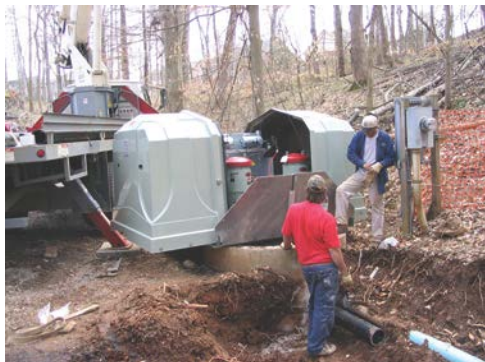
Figure 10: Installation Complete with Backfilling of Tied-In Force Main and Start-Up
