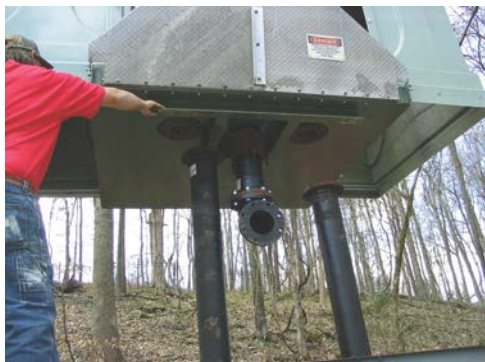
Figure 6: Commencing to Install Suction Pipes
