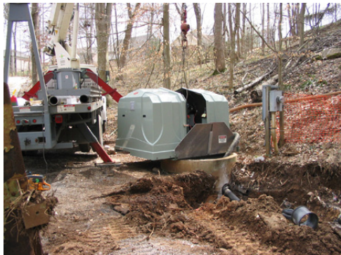
Figure 9: Awaiting Connection of Discharge
