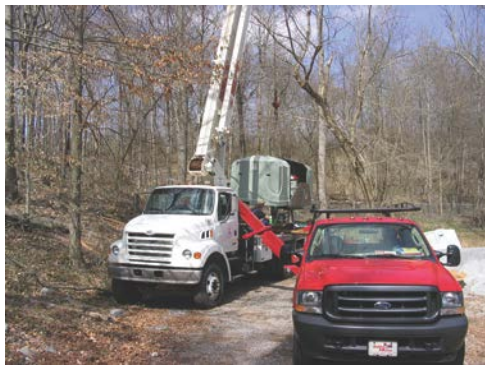
Figure 5: Lift Station Arrives at Job Site with Lift Truck for Installation
