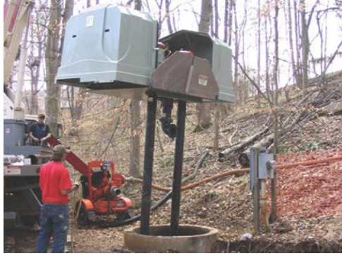
Figure 8: Placing Lift Station over Wet Well
