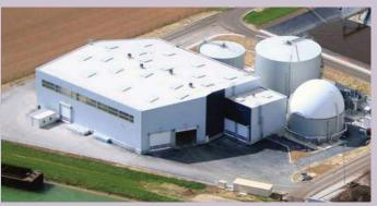
**BIOMET™** is an advanced anaerobic co-digestion process for the conversion of high strength and municipal organic waste to bioenergy and biofertilizer.
