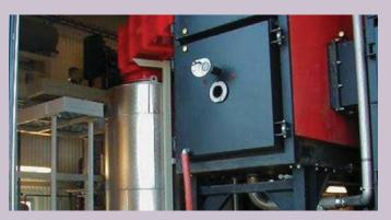
Additionally, the BioCon™ dryer can be fueled by the biosolids end product by incorporating the ERS which can result in an autogenous system by combusting the end product and utilizing the heat of combustion to fuel the dryer.
